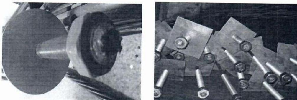
Figure 1 – Construction of a rope anchor
