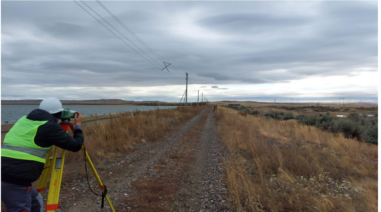
Figure 2 – Carrying out high-precision leveling of an earthen dam
