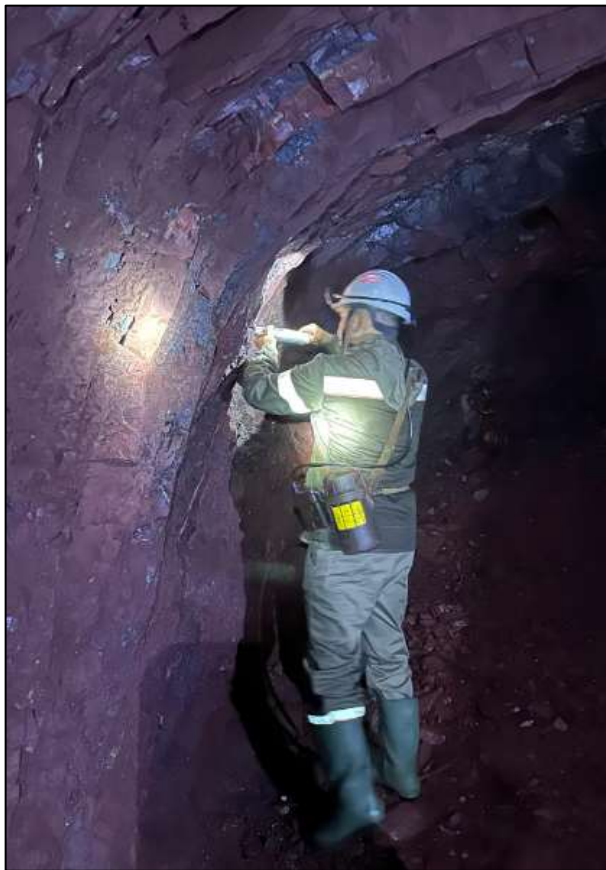
Figure 1 - Determination of intact rock strength (IRS) in mine workings using the Schmidt hammer
